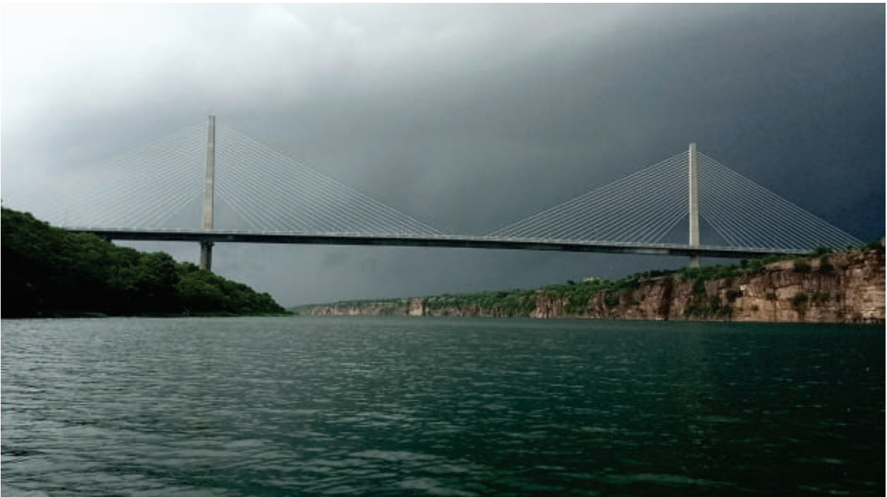
Figure 17. A view of cable-stayed bridge from Chambal River
